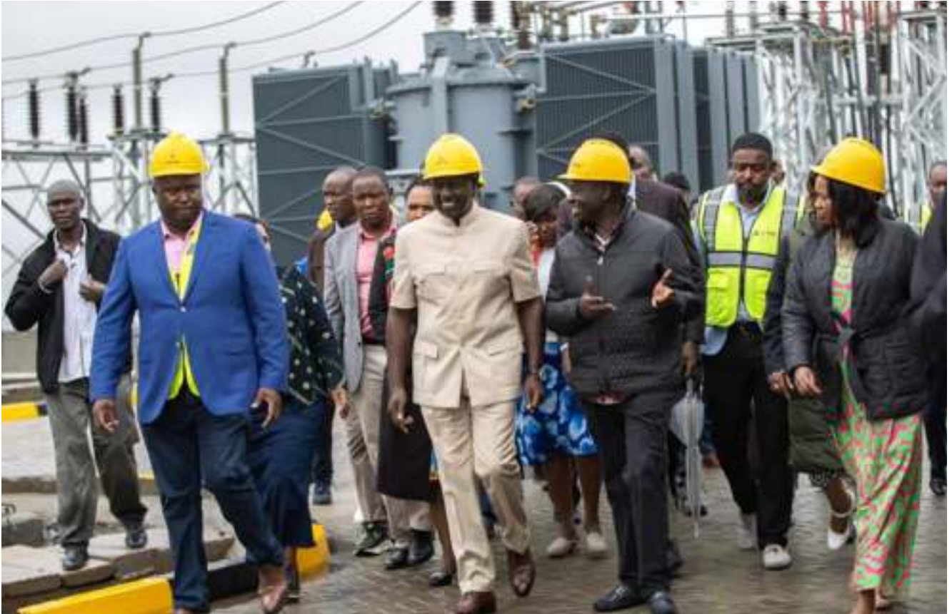
H.E President William Ruto and Deputy President Rigathi Gachagua during the commissioning of the Naivasha Special Economic Zone 900 MVA, 66/11KV Sub-station processes
